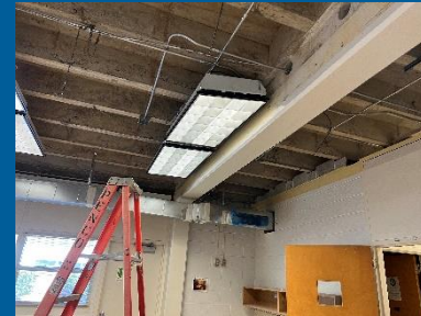
Installation of feeder conduit for VRF cassette unit in Area E
