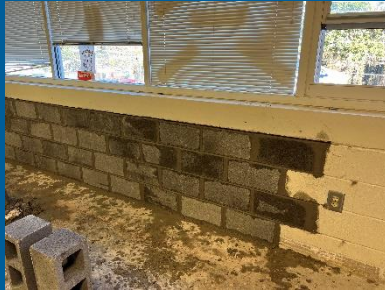
CMU infill at unit ventilator locations in Area D (West)
