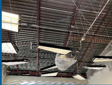
Rough-In of VRF cassette and piping in classroom of Area B
