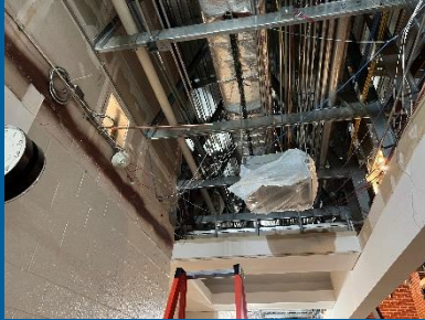
Rough-in of lineset piping to VRF unit in Area B
