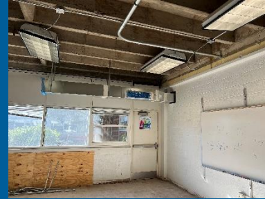
Block cut and rough-in of mechanical ductwork in Area D
