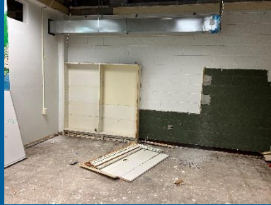
Selective demolition of casework in Area D
