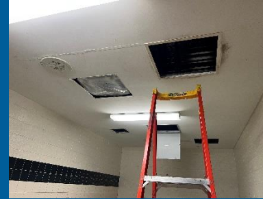
Installation of VRF cassette in ceiling of restroom in Area A
